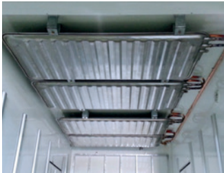
Eutectic plate Eutectic cold van HD45 ~ HD170 Material is STS 304 1.2t, and PCM-33°C solution is charged Note: Standard
